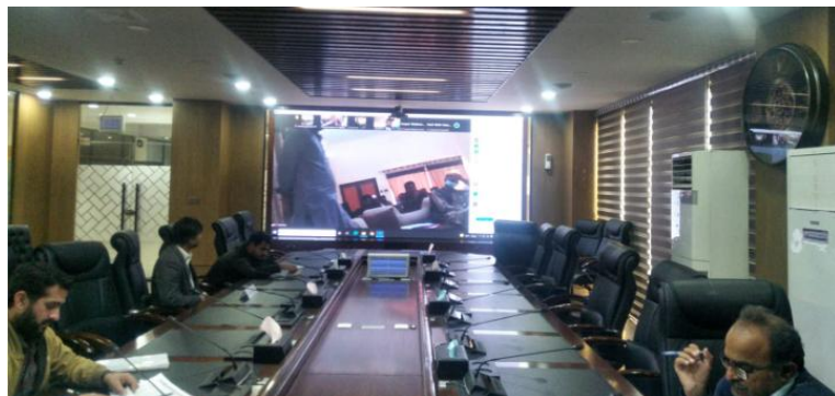
CENTRALIZED MONITORING AT N3C, PBS HEAD OFFICE
